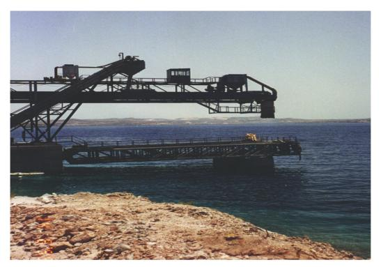
The loaders type JBM 500 are specific loaders for loading of dry, free flowing bulk materials onto ships.
